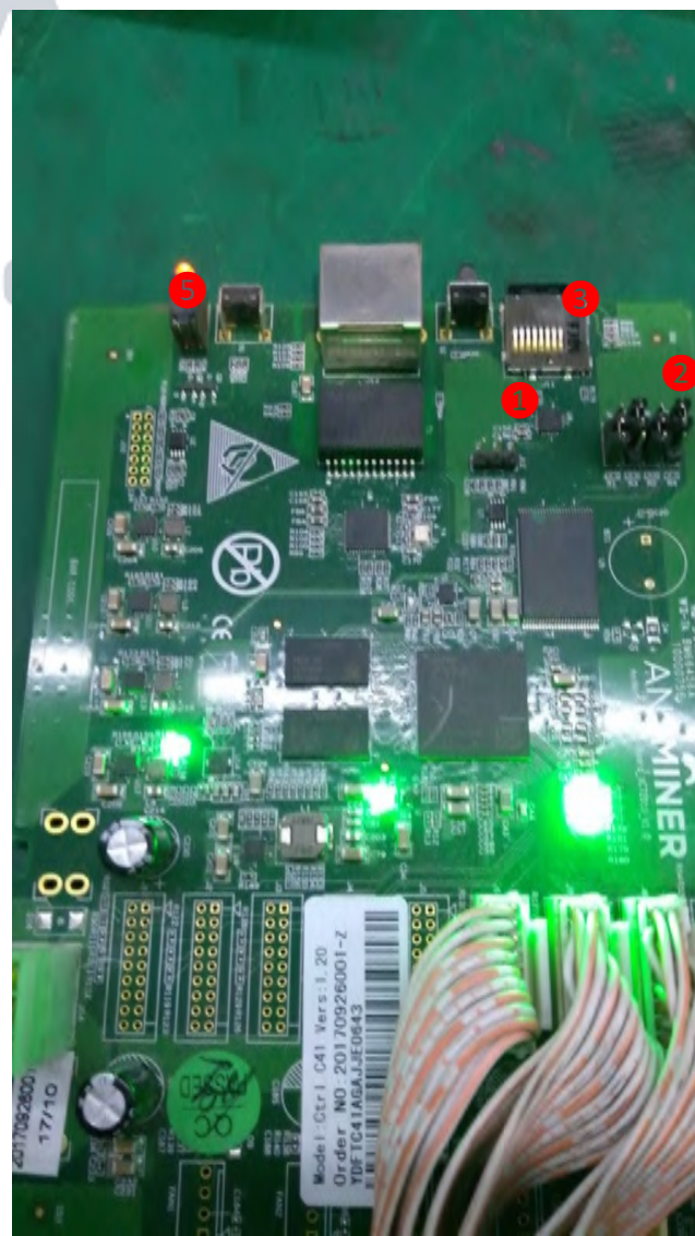
In the process of upgrade
